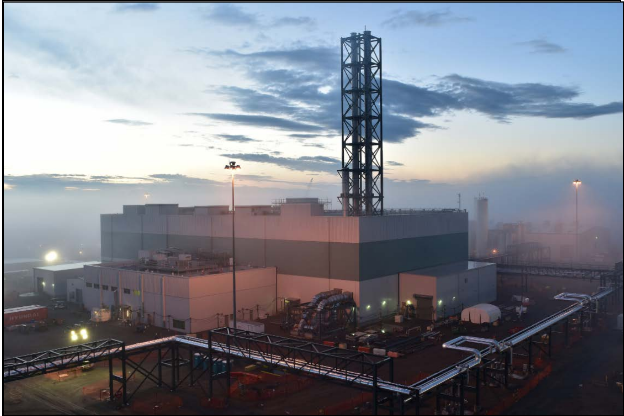
Fig. 2. Waste Treatment and Immobilization Plant Low-Activity Waste Facility.
